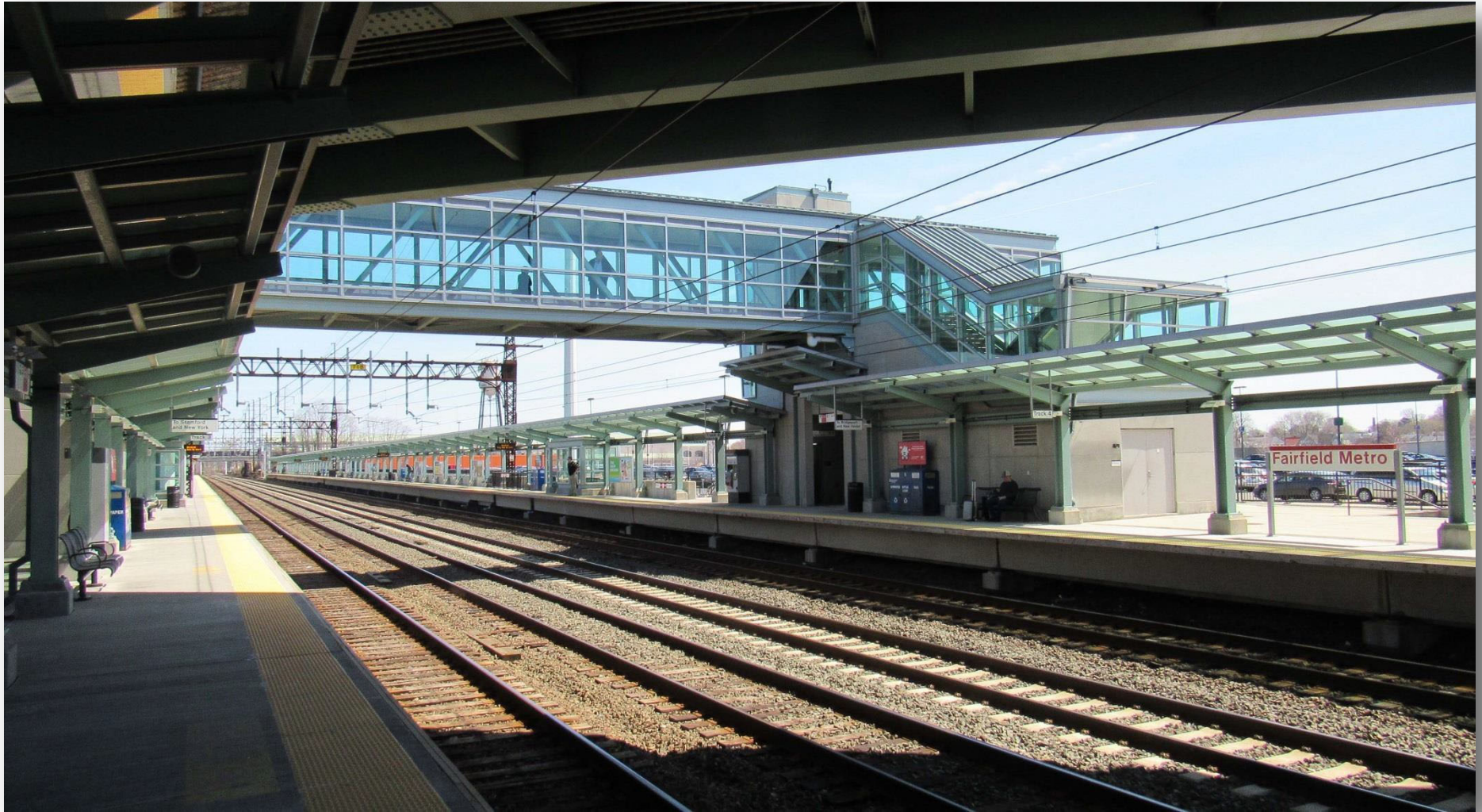
Metro North Train Station Platform Next Door
